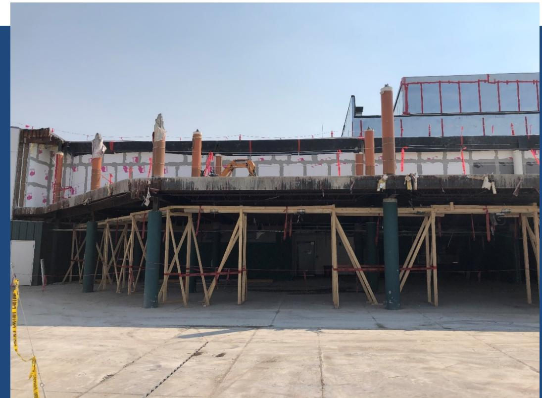
Wooden support structure holding up existing cold/hot water lines that are needed for the current HVAC system
