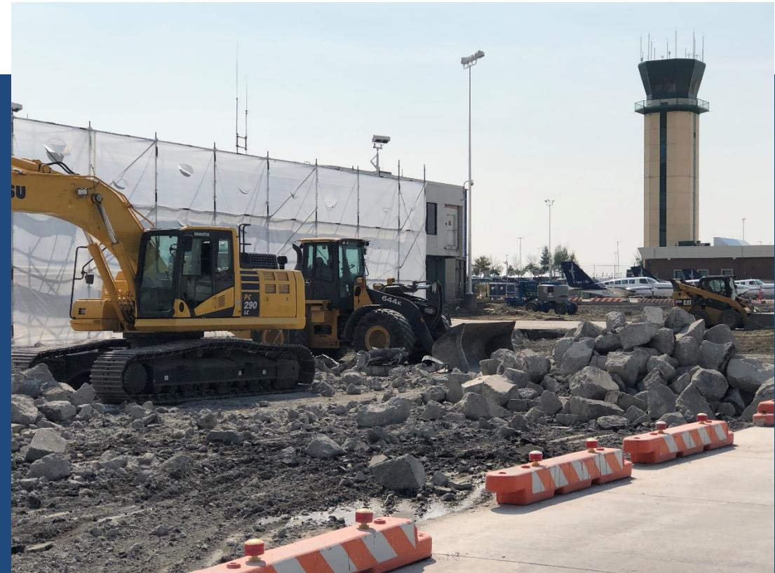
Removal of concrete aircraft parking ramp to make way for new TSA Screening Area, the Great Room, and A Concourse
