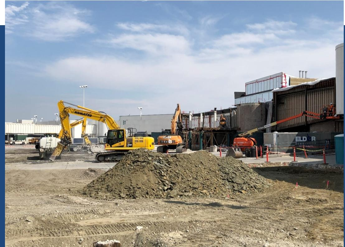
Utility work to install new underground electrical power, water and sewer service to new Concourse
