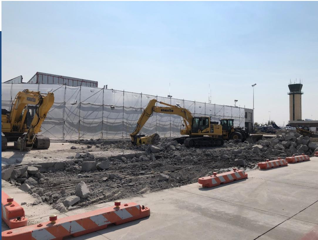
Protective barrier to keep debris, insulation, siding, roofing in work area, so it is not ingested into engines.
