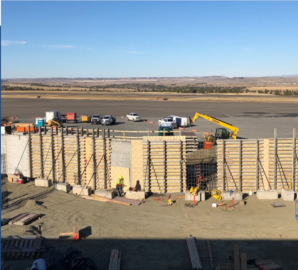
Setting large heated wall forms in place to pour concrete in cold weather.
