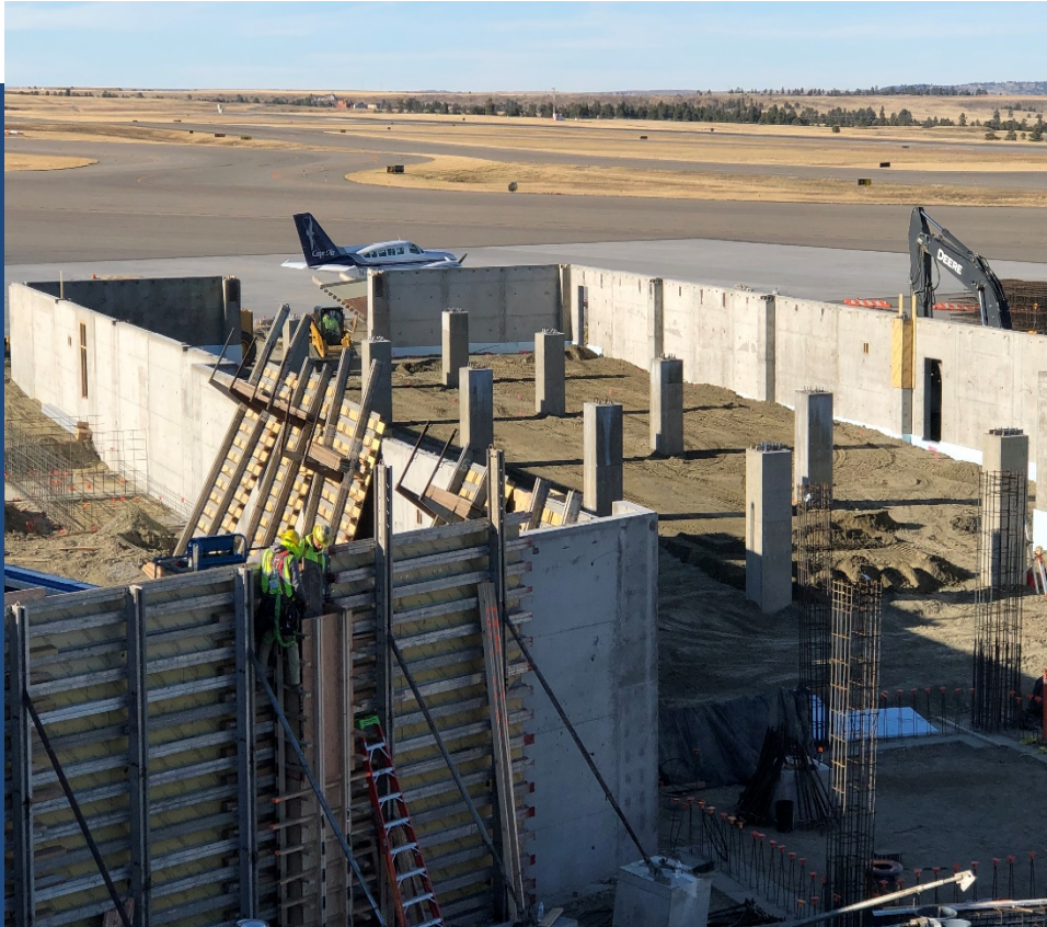
Forms are removed from new concrete foundation walls for new A Concourse.
