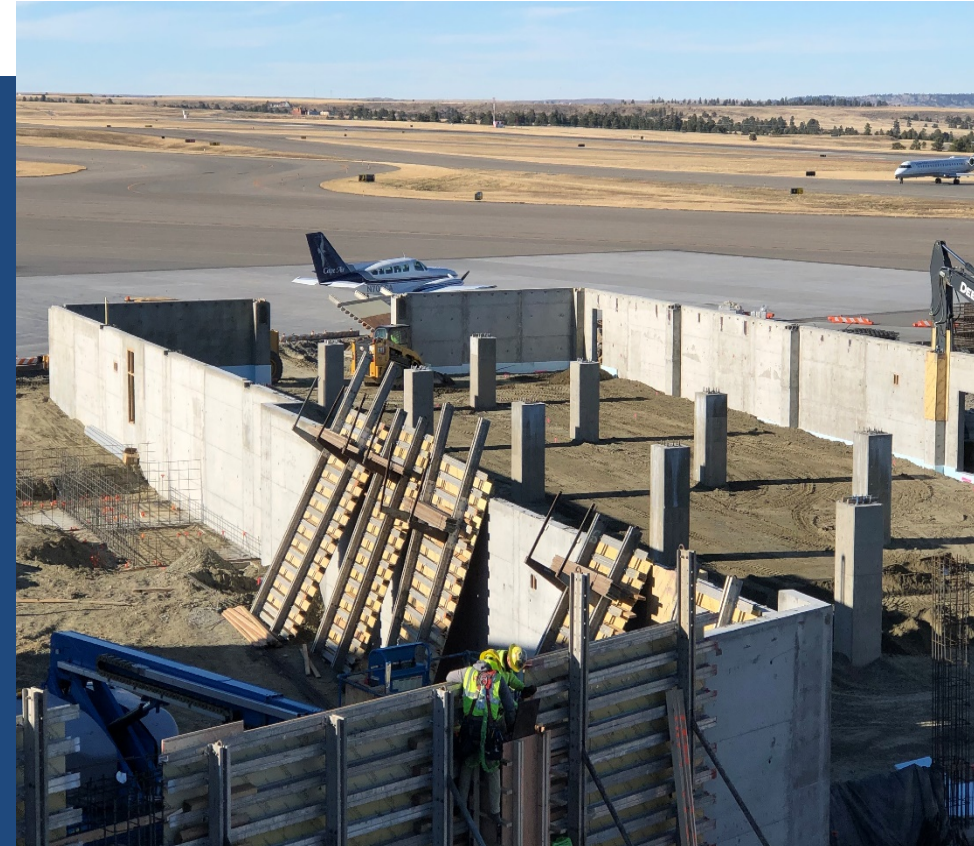
Concrete columns in place on northeast corner of the new A Concourse.
