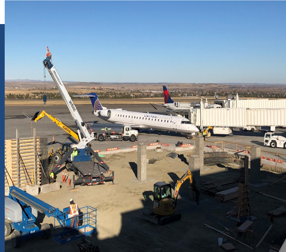
Steel rebar is set for concrete columns at northeast corner of the new A Concourse while flights continue to operate.
