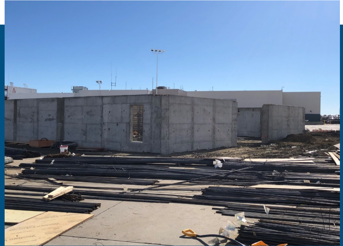
Massive amounts of steel rebar for the support columns on the northwest section of the new A Concourse.
