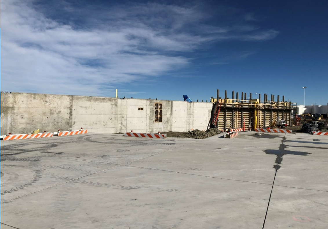
Special heated wall forms in place allowing concrete to be poured in cold weather.
