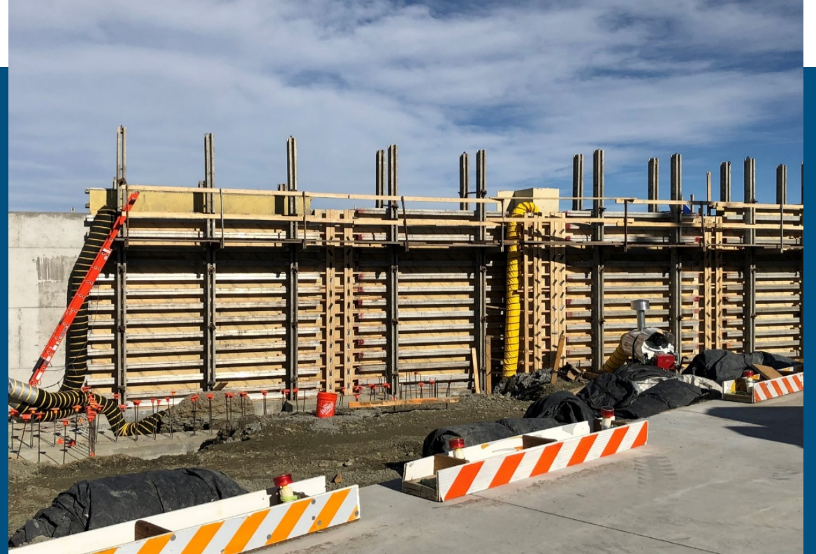
Close-up of special heated forms supporting the walls for the new A Concourse.
