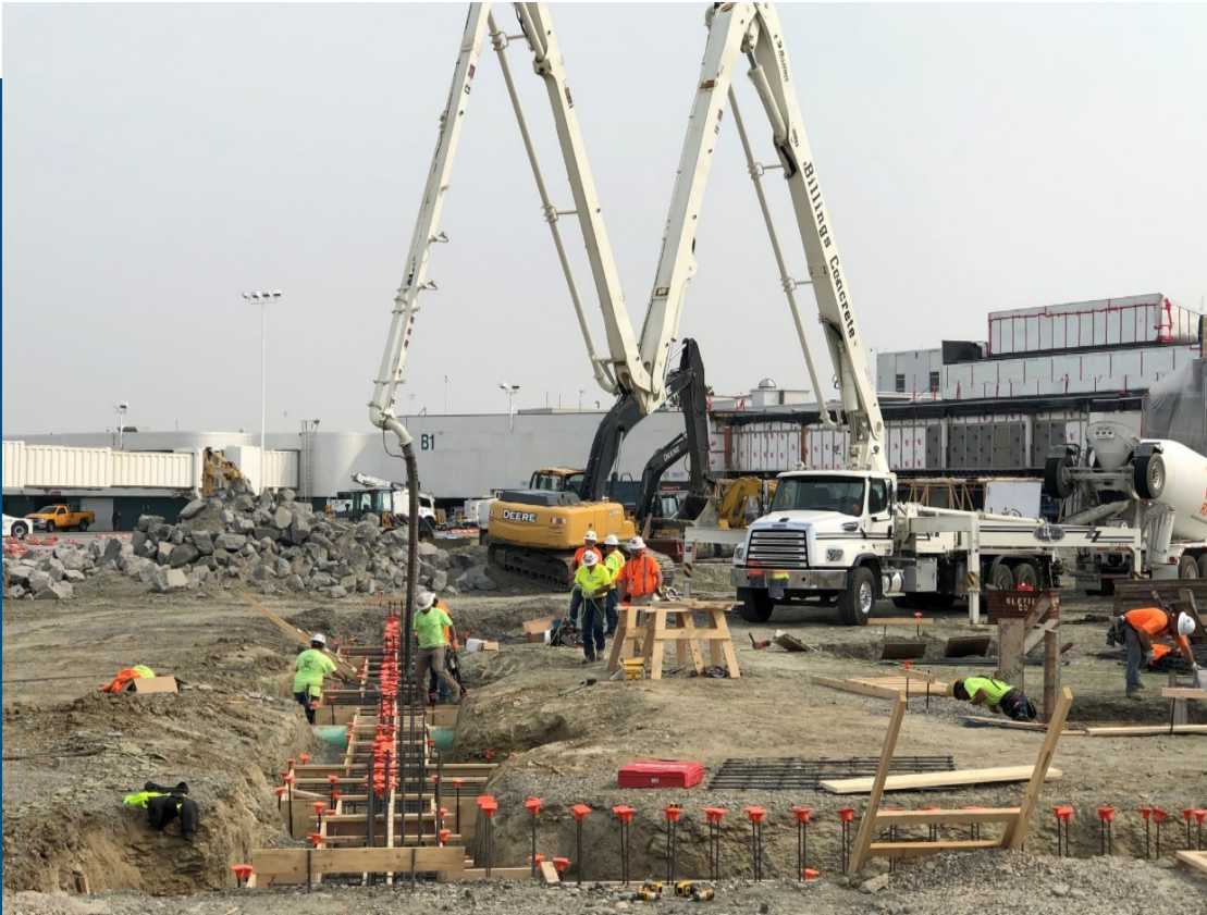
Construction crew pours new footings.
