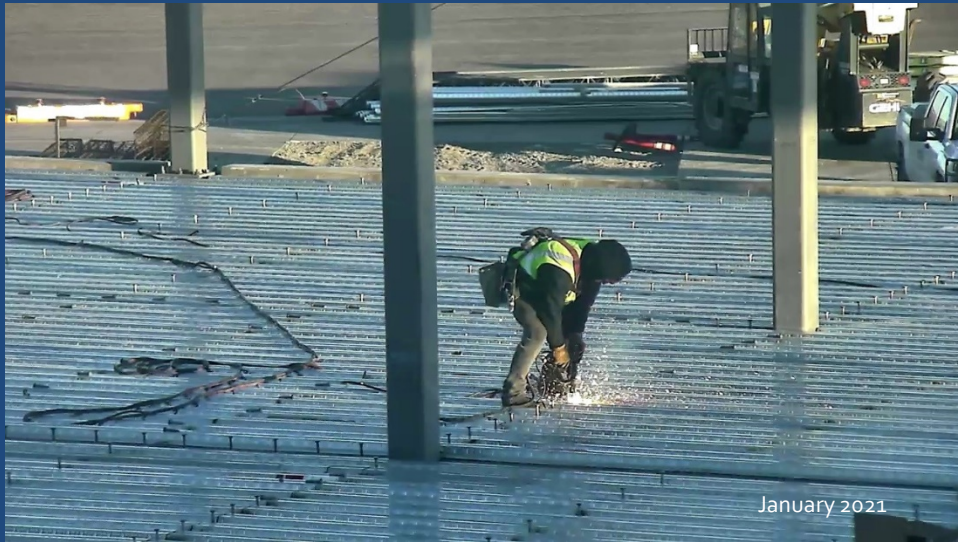
Steel bridge decking being pinned into place.
