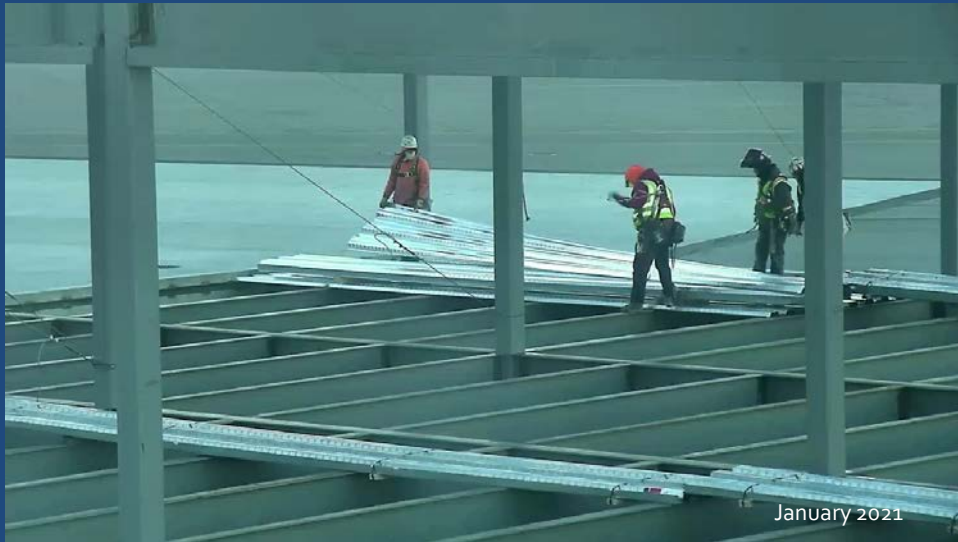
Steel bridge decking cover on floor.
