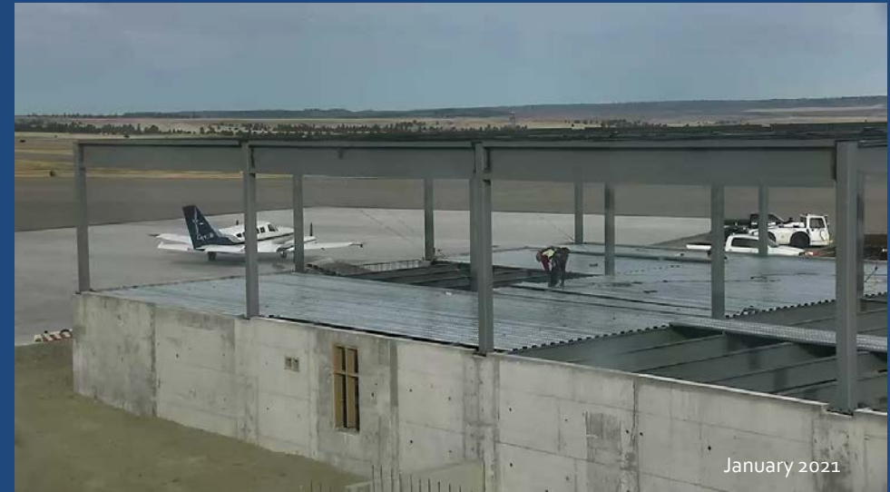
Steel bridge decking cover on floor.
