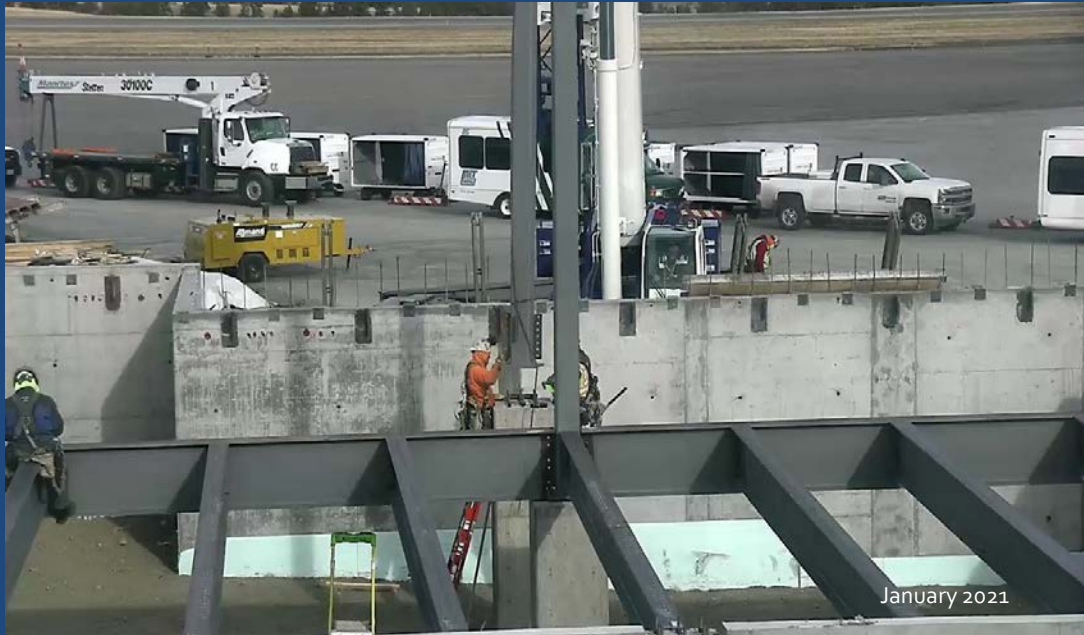
Steel beams for floor decking.
