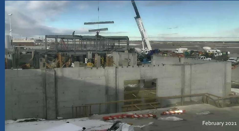
Steel I-beam installation and decking to support the new floor.
