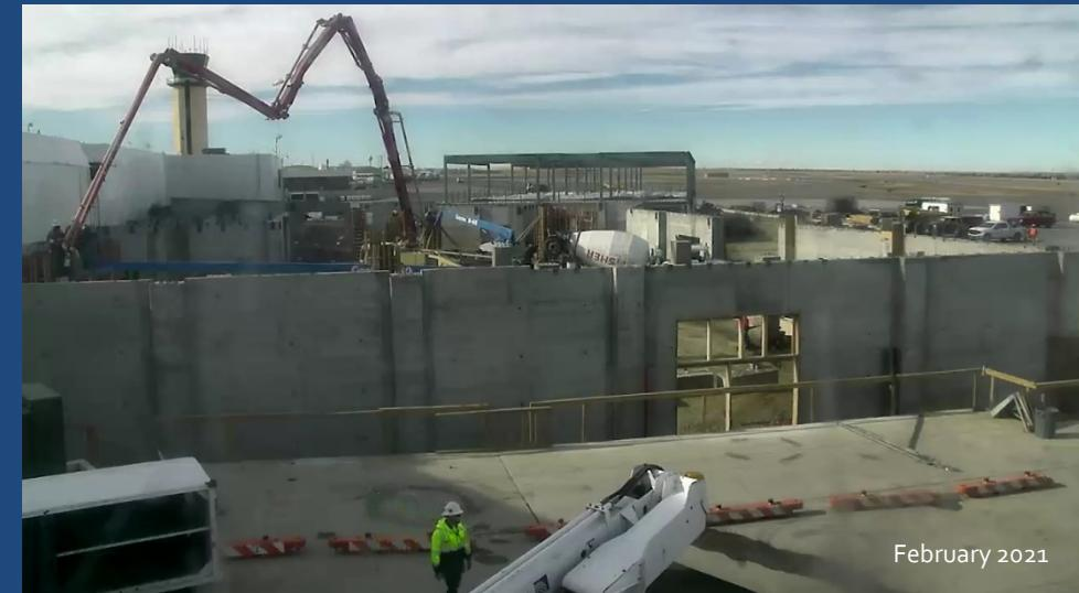
Concrete pump truck on interior wall pour.
