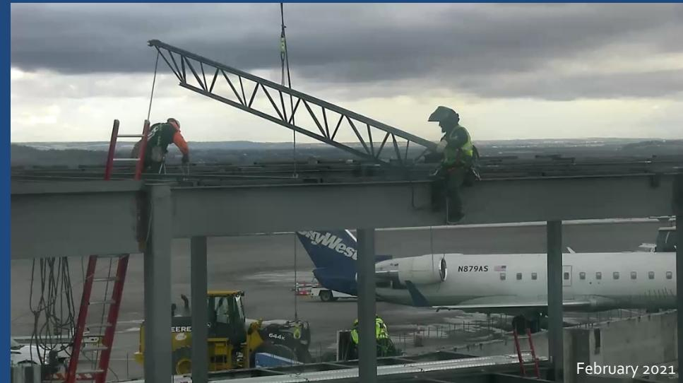
Steel truss installation continues to support the new roof structure.
