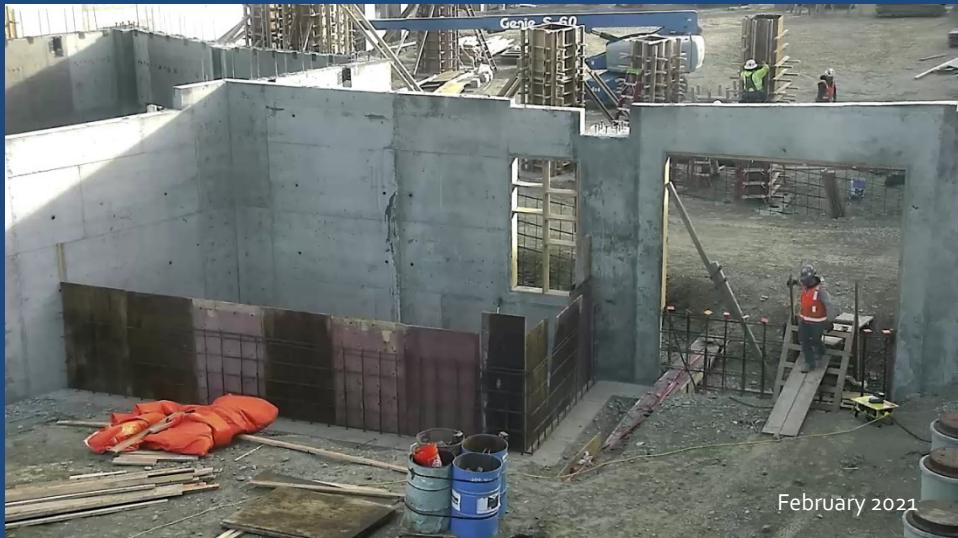
Setting forms to pour new concrete pad for new
