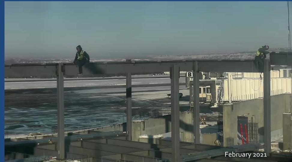
Steel beam placement continues to support the roof and skylight structure.
