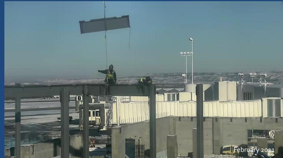
Steel beam placement to support the roof and skylight structure.
