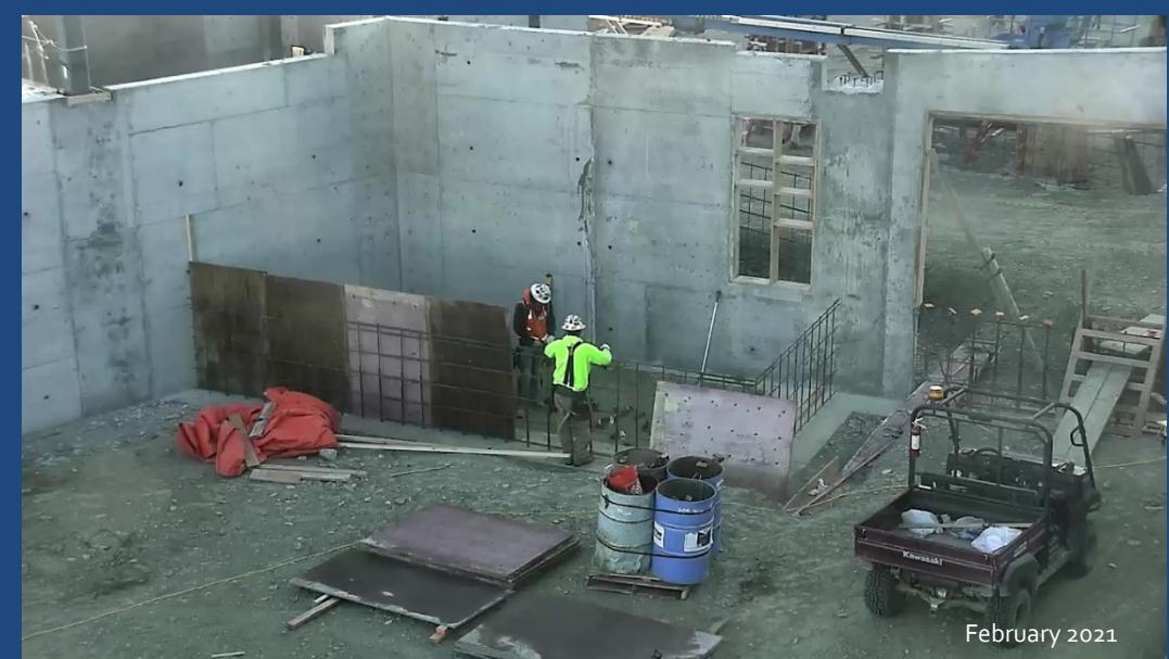
Setting forms to pour new concrete pad for new
