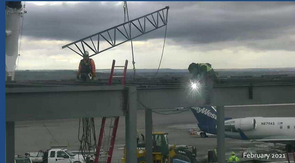
Steel trusses are installed to support the new roof structure.
