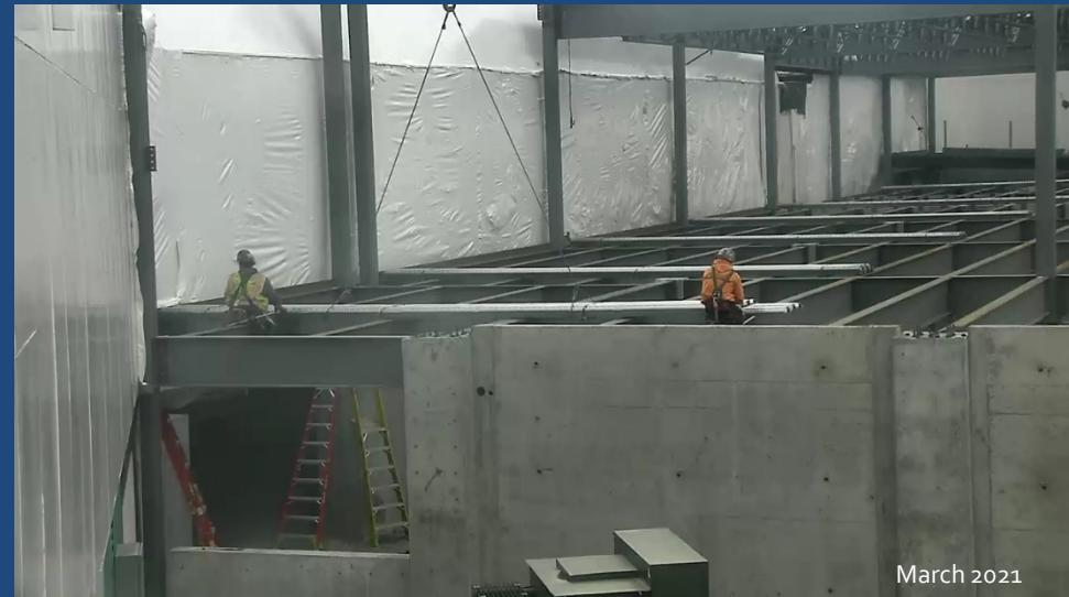
Sheets of steel are placed on I-beams to support the floor in the Great Room.
