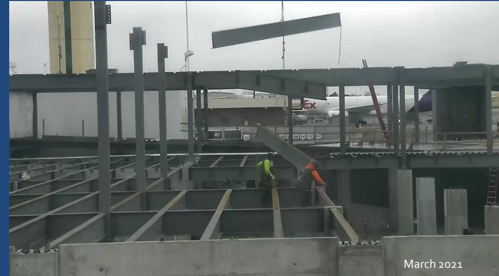
Heavy duty steel I-beam installation continues to support the walls and roof.
