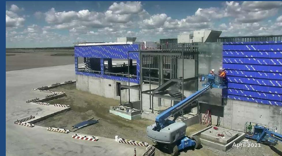
Steel panels are installed on the south stairwell and freight elevator.
