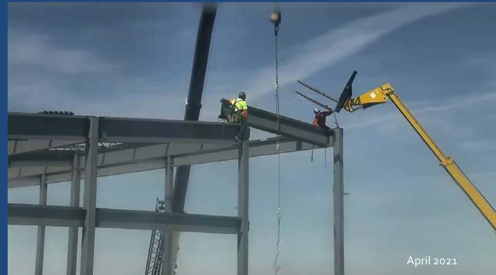
I-beam steel installation to support the roof structure.
