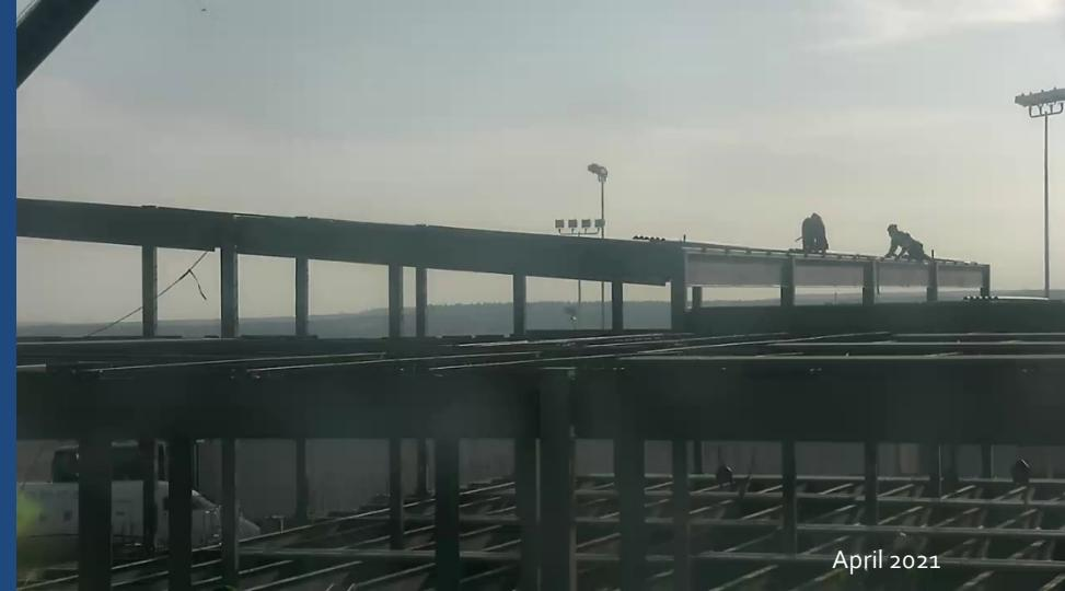
Steel decking installation to support the roof structure.
