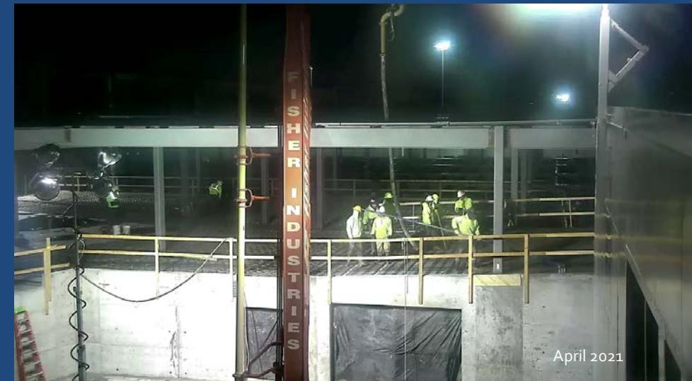
Pouring concrete for exit ramp to baggage claim.
