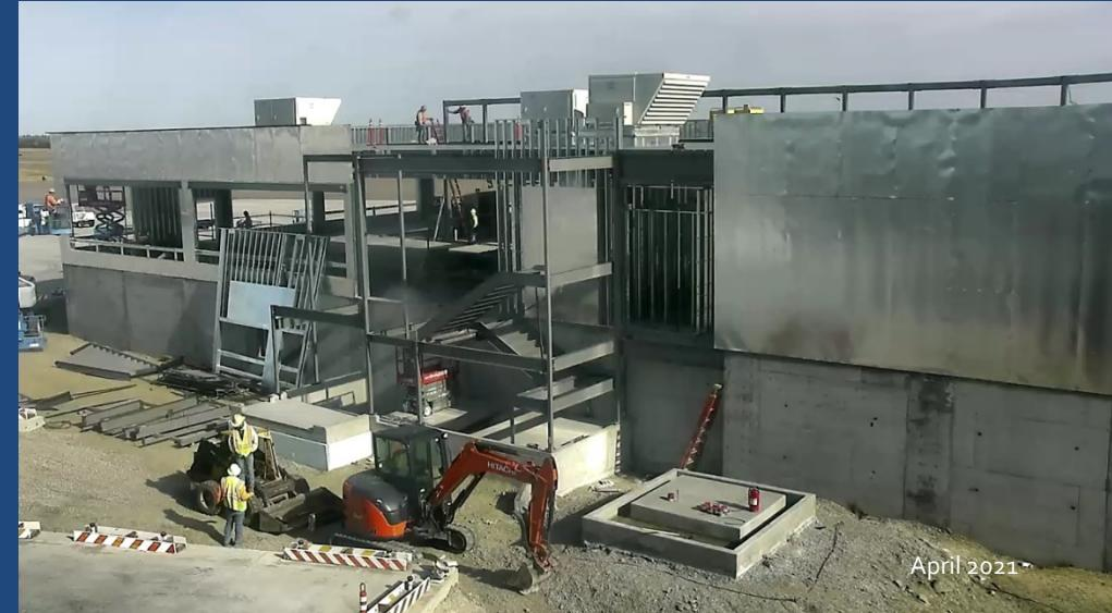
Exterior steel panels are being installed.
