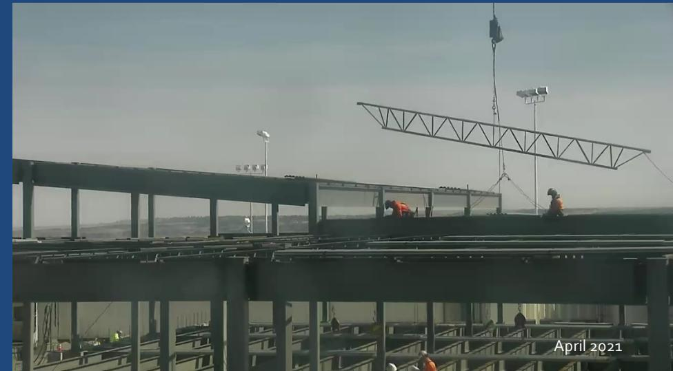
Setting ceiling trusses in place.
