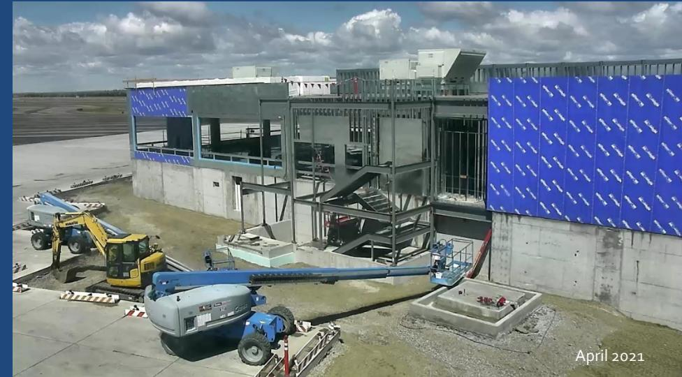
Steel panels and blue-skin cover are being installed on the south side of Concourse A.
