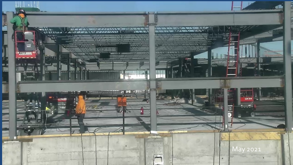
Erection of steel wall and roof support columns continued.
