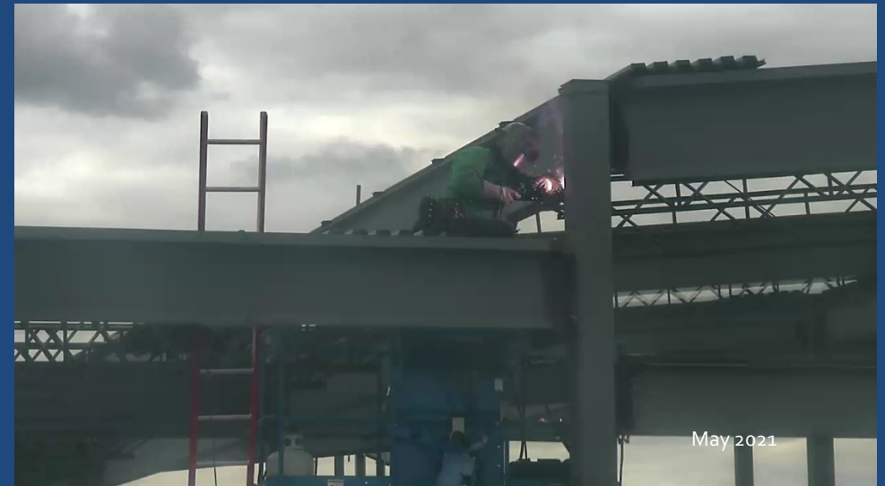
I-beam supports being welded in place.
