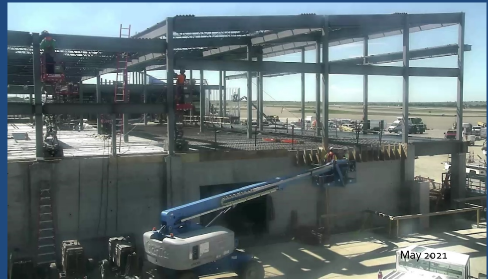
Steel erection of wall and roof support columns.
