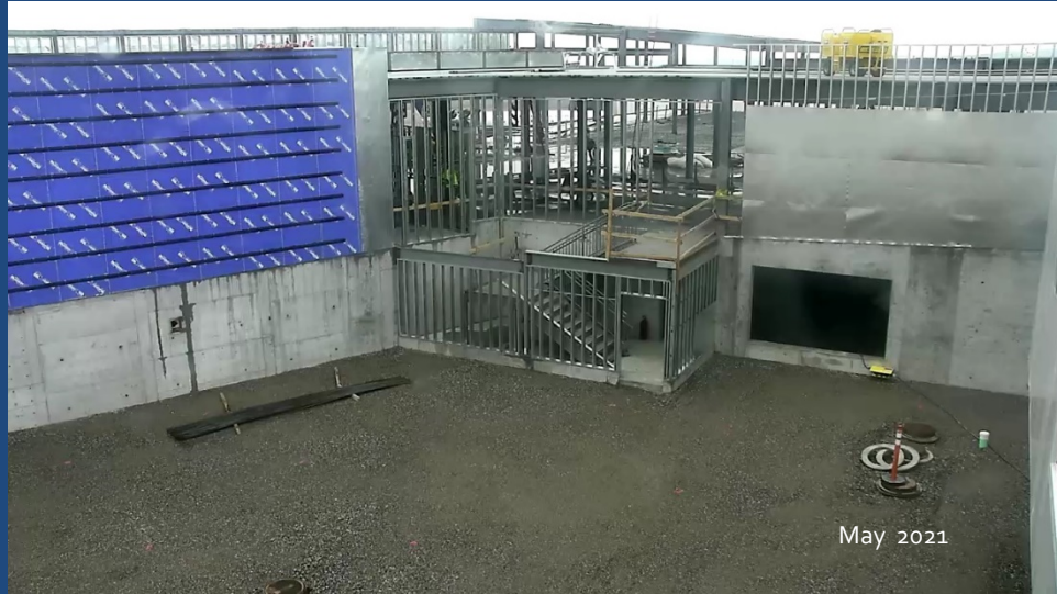
Steel framing of exterior stairwells.
