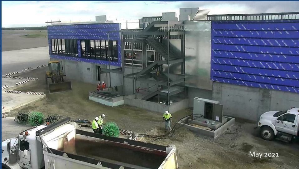
Utility work – installation of electrical transformer.
