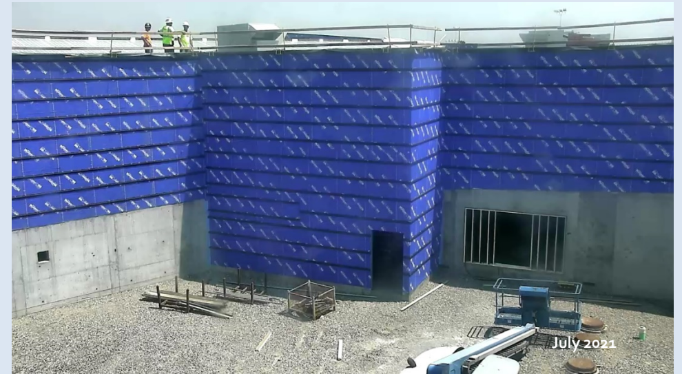
South view of Concourse A and new stairwells. Blue skin insulation and tracks for siding are being installed.
