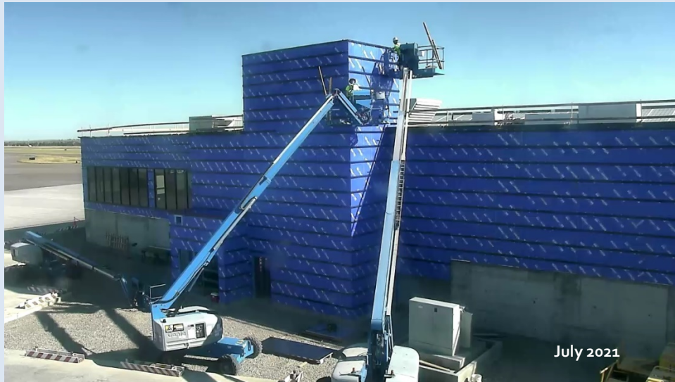
South view of Concourse A and new stairwells. Blue skin insulation and tracks for siding are being installed.
