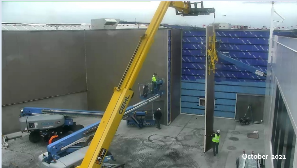
New siding panels being lifted into place.
