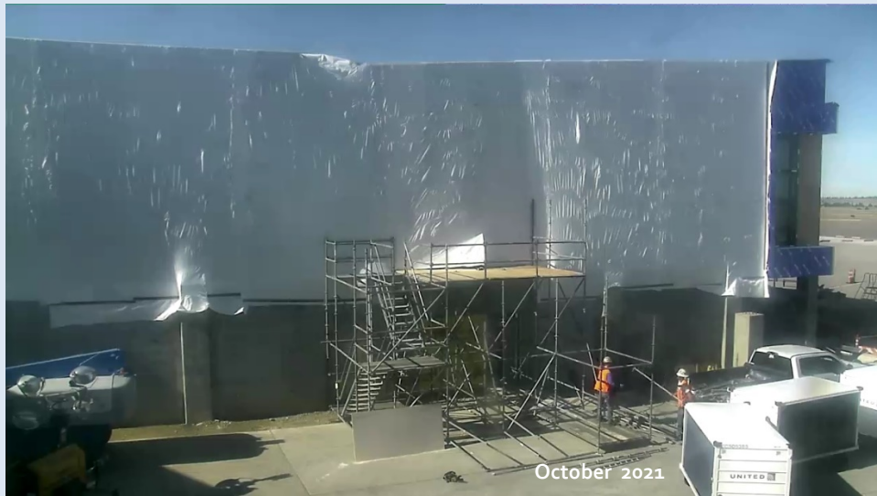
East wall of Great Room weatherproofing prior to Winter.
