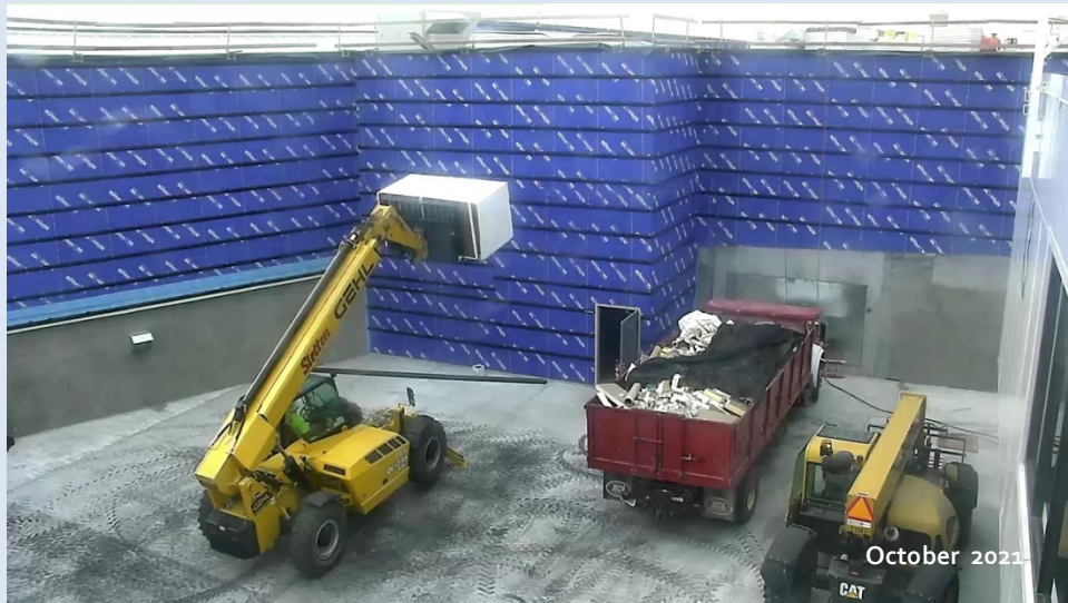
Roof work. Insulation panels being lifted into place.
