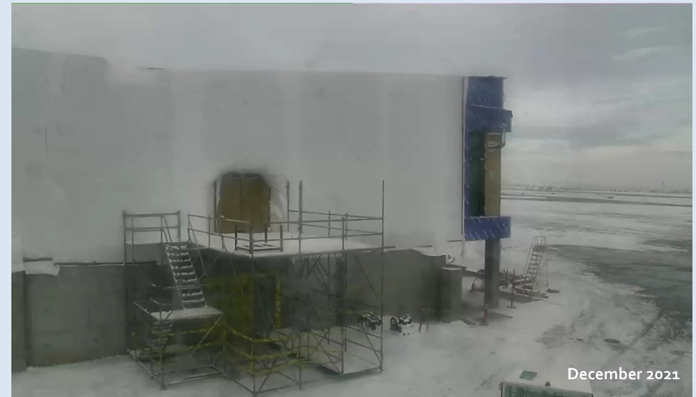
Weatherproofing of East wall of Great Room and scaffolding/temporary door for access.
